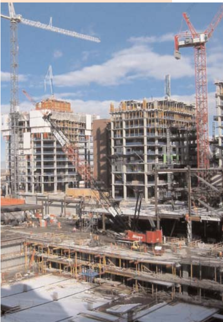
Winter 2009, Major construction seen from the window of our office.
