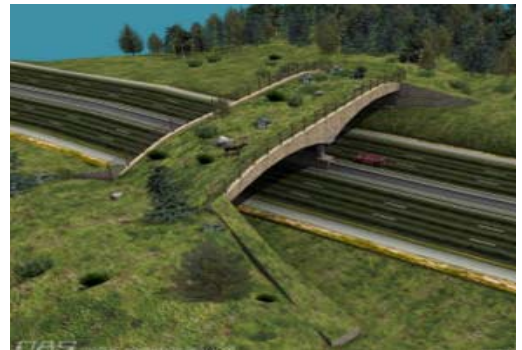
Artist's rendition of proposed wildlife overpass now being built over Interstate 70 near Vail pass in Colorado. Image courtesy of Center for Native Ecosystems
